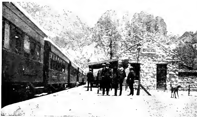
TRANSANDINE RAILWAY, USPALLATA STATION.
